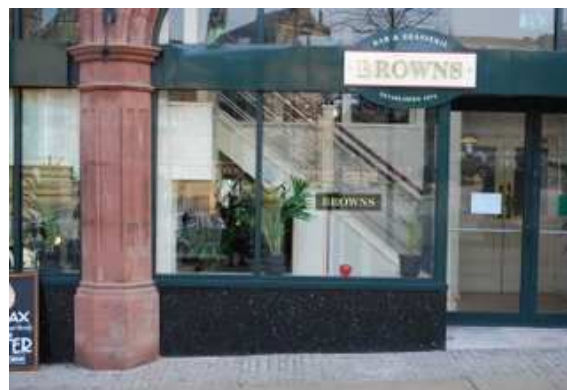
Building stones in a city centre – red sandstone and 'granite' make up the front of the café, whilst granites and buff sandstones form the paving. St Paul's Parade, Sheffield (Photo: Peter Kennett )
