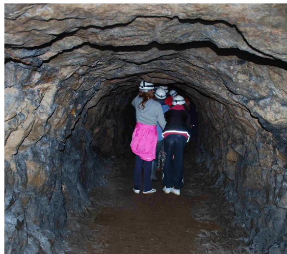
An unsupported tunnel in limestone, dug by copper miners in 1804 (All photos: Peter Kennett )
