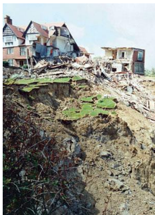
Holbeck Hall Hotel, Scarborough, Yorkshire, kollapset i 1993. (BGS photo ID 10741/1).
