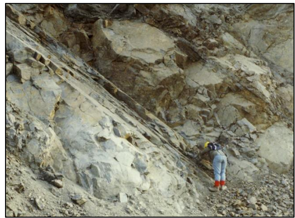
Overhanging rocks, Dolyhir Quarry, Wales, UK
