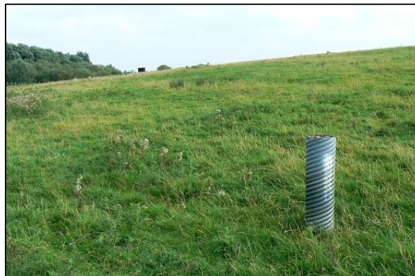
Vent to release potentially dangerous methane from landfill filling an old quarry, Severn Way, near Hempsted, Gloucestershire, UK.
