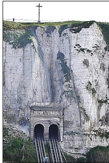
Railway tunnel into a chalk cliff, Le Treport, Normandy, France.
