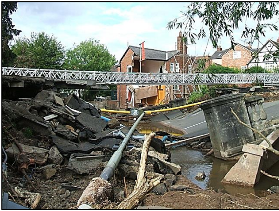
Burway Bridge over the River Corve, Ludlow, England after the floods.
