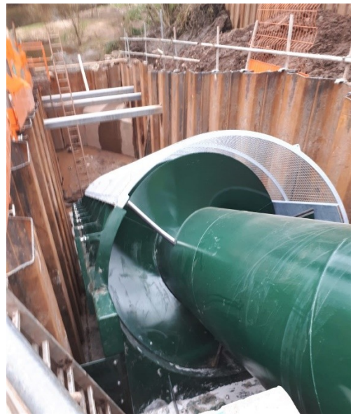
The River Dane Archimedes screw under construction (March 2021. Photo: Peter Lane)
