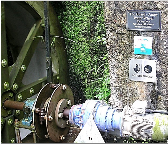
Close up of the generator at the Forest of Dean (Photo: P. Kennett)
