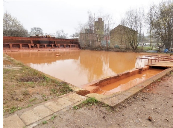
A settling tank for warm mine water pumped out of workings at the National Coal Mining Museum, near Wakefield, Yorkshire. (© Copyright Stephen Craven and licensed for reuse under this Creative Commons Licence.)
