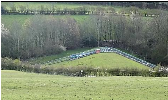
A dam designed to hold back flood water and then release it in a controlled way. Dronfield, near Sheffield
