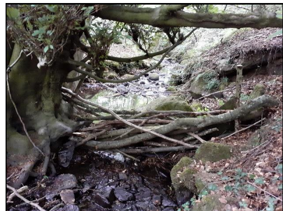
A 'leaky dam' constructed by volunteers
