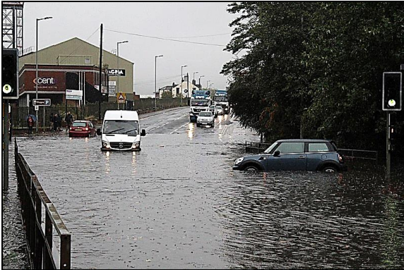
Flooding in the Don Valley, South Yorkshire.
