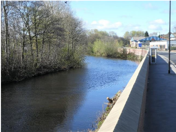
Newly raised walls 2m high alongside the River Don at Meadowhall.
