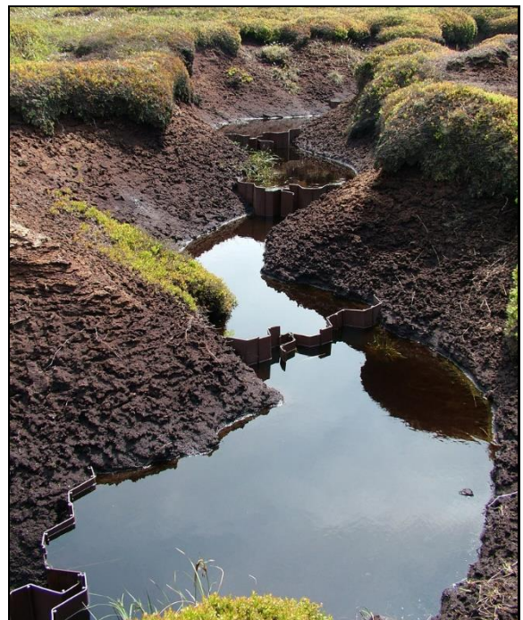
Plastic mini dams in a peat bog to hold back water to promote moss growth.
