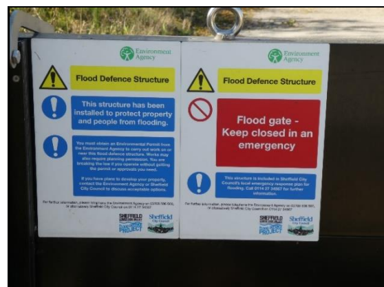
A flood barrier between the River Don and the main road, which can be opened or shut as required.
