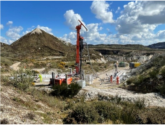
A drilling rig prospecting for lithium in a former china clay pit in Cornwall ( www.businesscornwall.co.uk/news )
