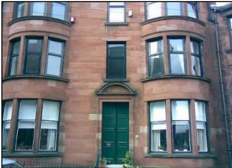
Building made of rock blocks - South side Glasgow Tenement (Shawlands) © George Rob
