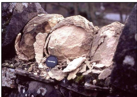
The effects of freeze/thaw weathering in a porous limestone. (Peter Kennett)
