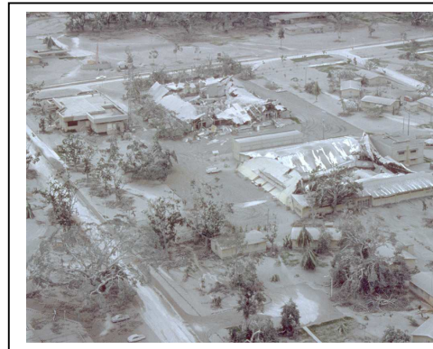
Aerial view of part of Clark Air Base, Luzon Island, the Philippines. Buildings and vegetation were damaged by ash fall from the eruption of Mt Pinatubo on 15 June, 1991.
