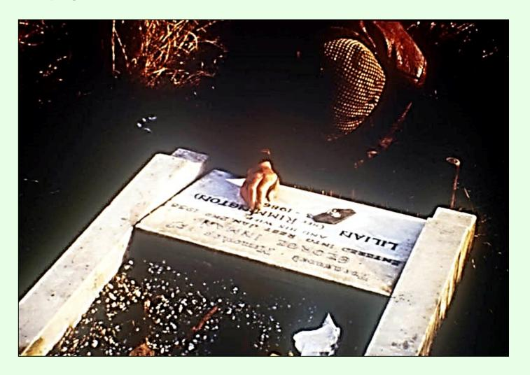
The mason adding a new name to a weathered marble slab
